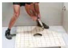
**4.** Once the plumbing & the flange have been installed, place the ProFinish™ tray back into position, use a sharp knife to cut around the outside of the waste flange until the tray fits neatly around the waste flange outer perimeter.
