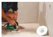
**1.** Before you begin, make sure the floor is clean, free of dust and is a level flat surface. Check using a spirit level and, if necessary, use a suitable levelling compound to correct any unevenness in the floor. When fitting the tray to a timber floor we recommend the use of a slate and tile underlay, particularly when the wooden floor has been oiled.
