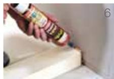
**6.** Ensure adhesive is applied to the sill ends - providing sill to wall joint adhesion.
