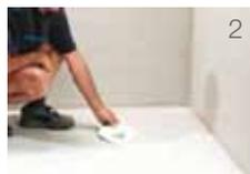
**2.** Place the ProFinish™ tray in position against the lined wall and mark the external perimeter of the tray and position of the waste flange with a pencil.
