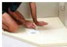
**3.** Remove the tray and fit the waste flange to the outlet in the floor.
