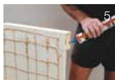
**5.** Lift the base and apply the adhesive supplied within the marked tray perimeter, using a 60mm grid pattern commencing 25mm in from the outer edges.
