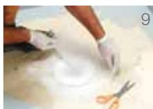
**9.** Apply the waterproof membrane according to the manufacturer's instruction. Ensure waterproofing is applied down into the waste flange and up the inside vertical face of the tile sill (hob), across the top edge and down to the floor line on the outside of the ProFinish™ tray. Where frameless doors are to be fitted it is recommended that floor areas outside the shower should also have a waterproofing membrane applied, prior to tiling.
